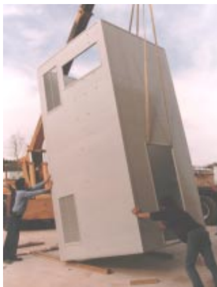
Above: Test facility fabricated of EXTREN ® , DURASHIELD ® , and FIBREBOLT ® for Compaq Computer Corporation. Left: All-fiberglass buildings constructed of DURASHIELD ® foam core panels and EXTREN ® fiberglass structural shapes are used to house communications, electrical, pumping or other equipment.
