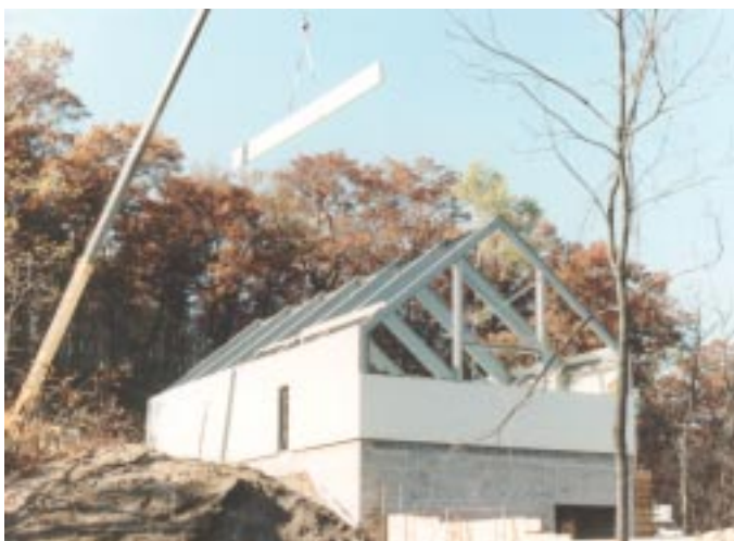
Above: This all-fiberglass facility for Amador Corp. assures RFI/EMI compliance in testing computers as well as other manufactured equipment.
