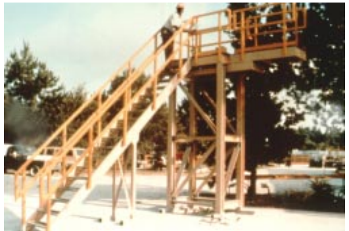
Above: All fiberglass tank car loading platform is a special cantilevered design.
