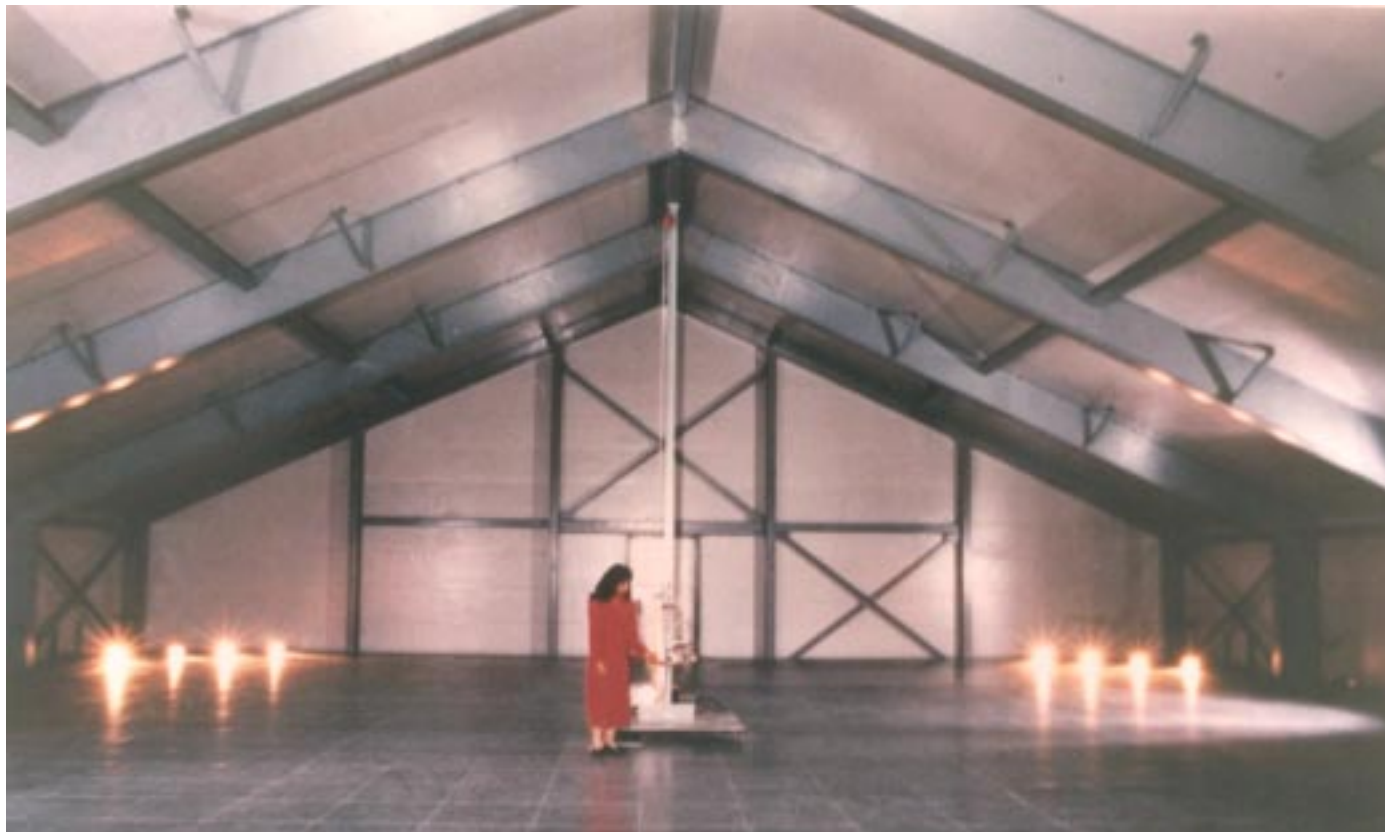
Above: Test facility fabricated of EXTREN ® , DURASHIELD ® , and FIBREBOLT ® for Compaq Computer Corporation. Left: All-fiberglass buildings constructed of DURASHIELD ® foam core panels and EXTREN ® fiberglass structural shapes are used to house communications, electrical, pumping or other equipment.
