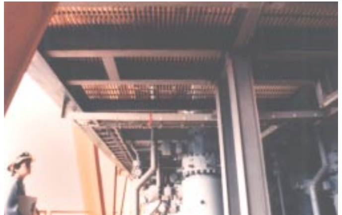
Above: This Well Bay Platform was easy to install requiring no heavy equipment, cutting torches or welding to make field modifications, thereby saving the cost of shutting wells down.
