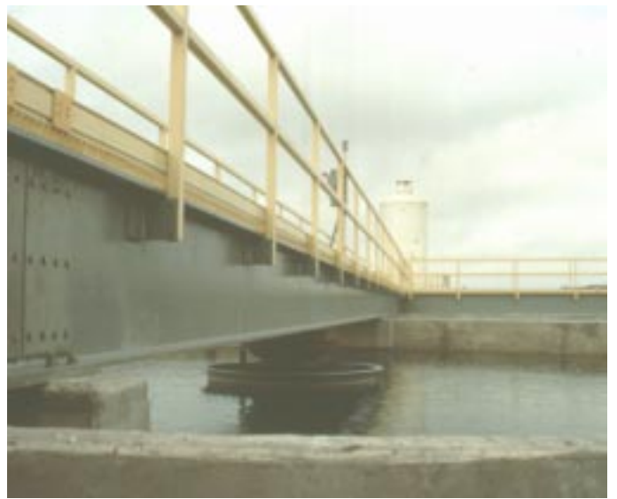
Above: Lightweight, corrosion resistant 24" fiberglass I-beams span 45' to bridge clarifiers at the Las Rusias, Texas Waste Water Treatment Plant. Left: 2500 feet of handrail was installed at the Fort Kamehameha Wastewater Treatment Facility, Pearl Harbor Naval Base in Hawaii.
