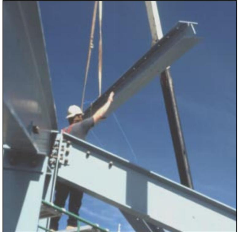
*Photo above: What you see here is not the erection of a steel structure. It is a structure being assembled using EXTREN® fiberglass structural members. Today, EXTREN® is replacing steel in a wide variety of structural applications. Why? Because EXTREN® is a problem solving material.*
