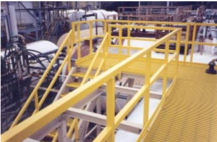
158 lineal feet of SAFRAIL™ handrail is used on this floating dock over corrosive effluent in a landfill seepage containment pit.
