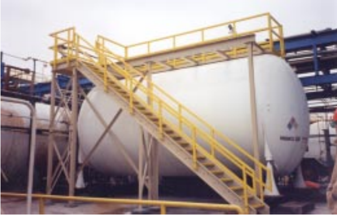
SAFRAIL™ system in a chemical plant.
