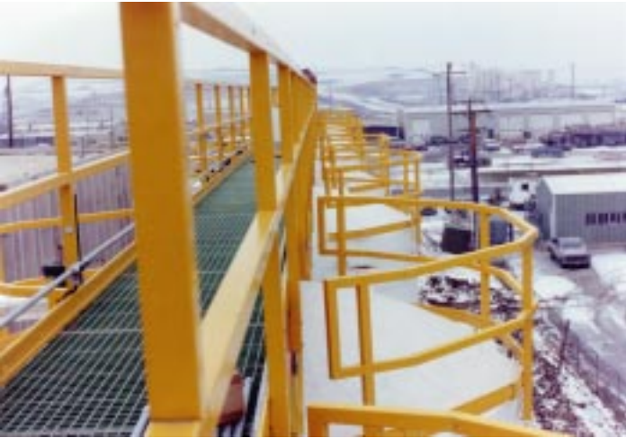
Internal connections make circular handrail systems such as these possible around tanks.
