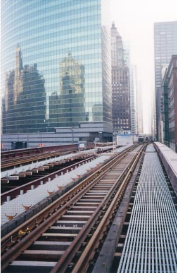
Above: Chicago Transit maintenance walkways alongside elevated train tracks constitute one of the largest fiberglass grating installations in history. This project used DURAGRID® T-5000 2" with a custom polyester resin.
