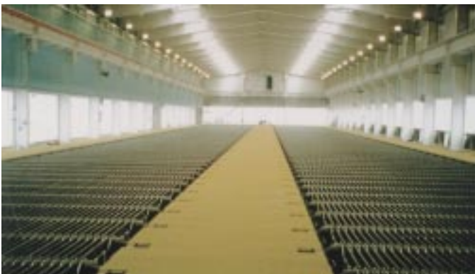
Above: Copper processing facilities such as the Ammonia Leach/Solvent Extraction/Electrowinning plant for Minera Escondida Limitada in Chile found DURADEK® I-6000 1-1/2" to be the perfect solution.
