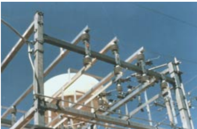
Nonconductive feeder beams made of EXTREN® prevent power outages.
