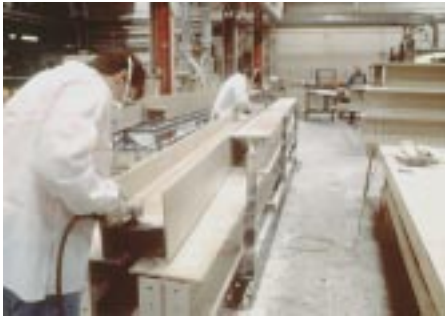
Beams are prepped before bonding connections together.
