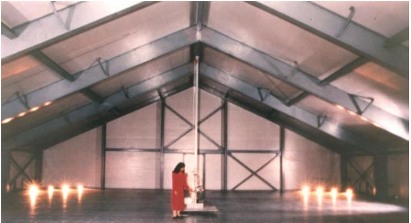
Above: 24" EXTREN® fiberglass I-beams span 62' wide rigid gables that support siding and roof of an all-fiberglass building used for computer testing.
