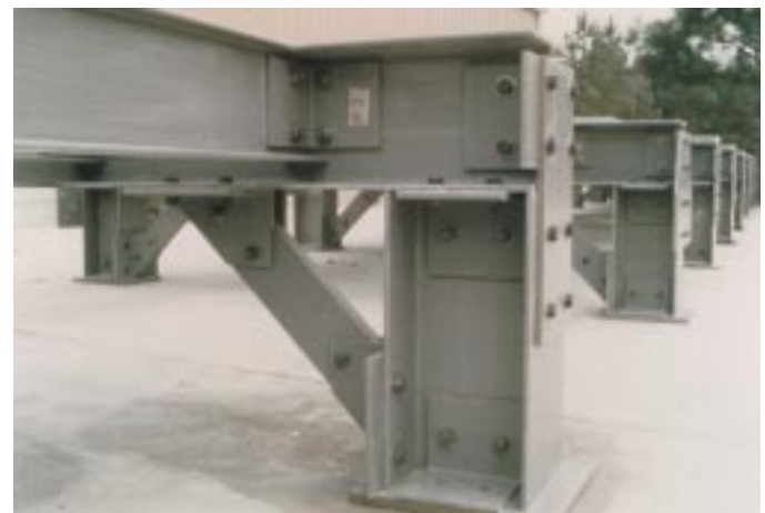
10' x 250' EXTREN® platform for a petrochemical complex.
