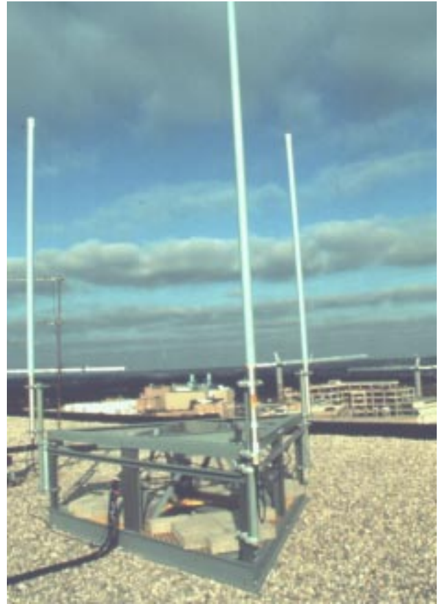
Lightweight and RFI/EMI transparent, EXTREN® provides support structures for Cellular One of Ohio antennae installed on building roofs and towers.
