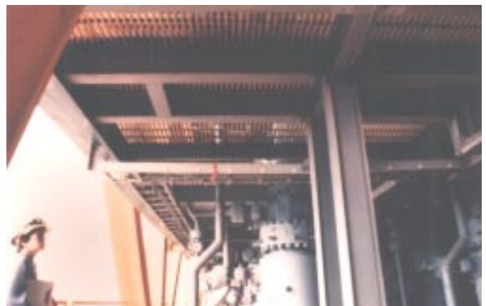
This Well Bay Platform was easy to install requiring no heavy equipment, cutting torches or welding to make field modifications, thereby saving the cost of shutting wells down.
