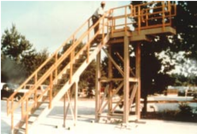
Below: All-fiberglass tank loading platform uses multiple EXTREN® sections.
