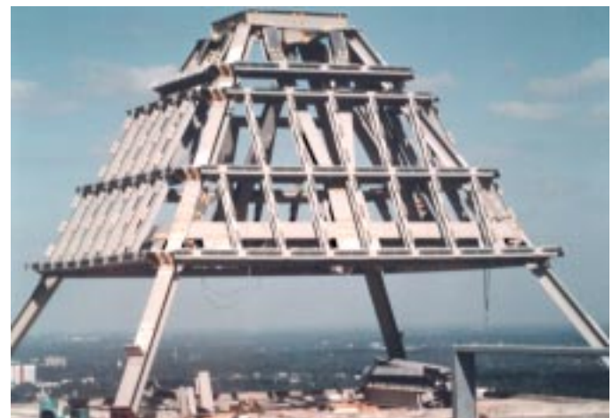
One of four three-story turrets constructed of EXTREN® to house communications equipment atop the Sun Bank building in Orlando, Florida.
