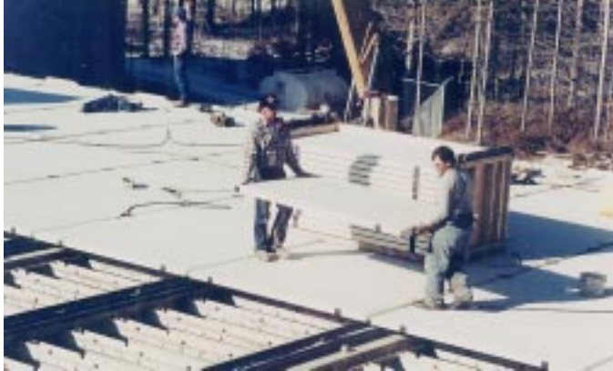
DURASHIELD® panels are used as plant roofs and chemical tank covers in corrosive environments, such as the covers (16,800 s.f.) over anaerobic digester units pictures above.
