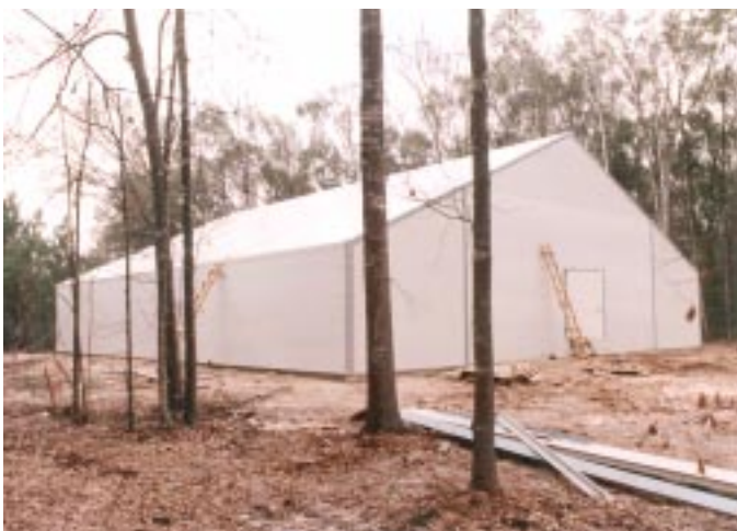
Compaq Computer chose a foam core panel building to assure RFI/EMI compliance for attenuation.
