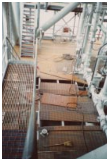
Above: DURAGRID® Phenolic grating for off loading platforms saves weight and maintenance.
